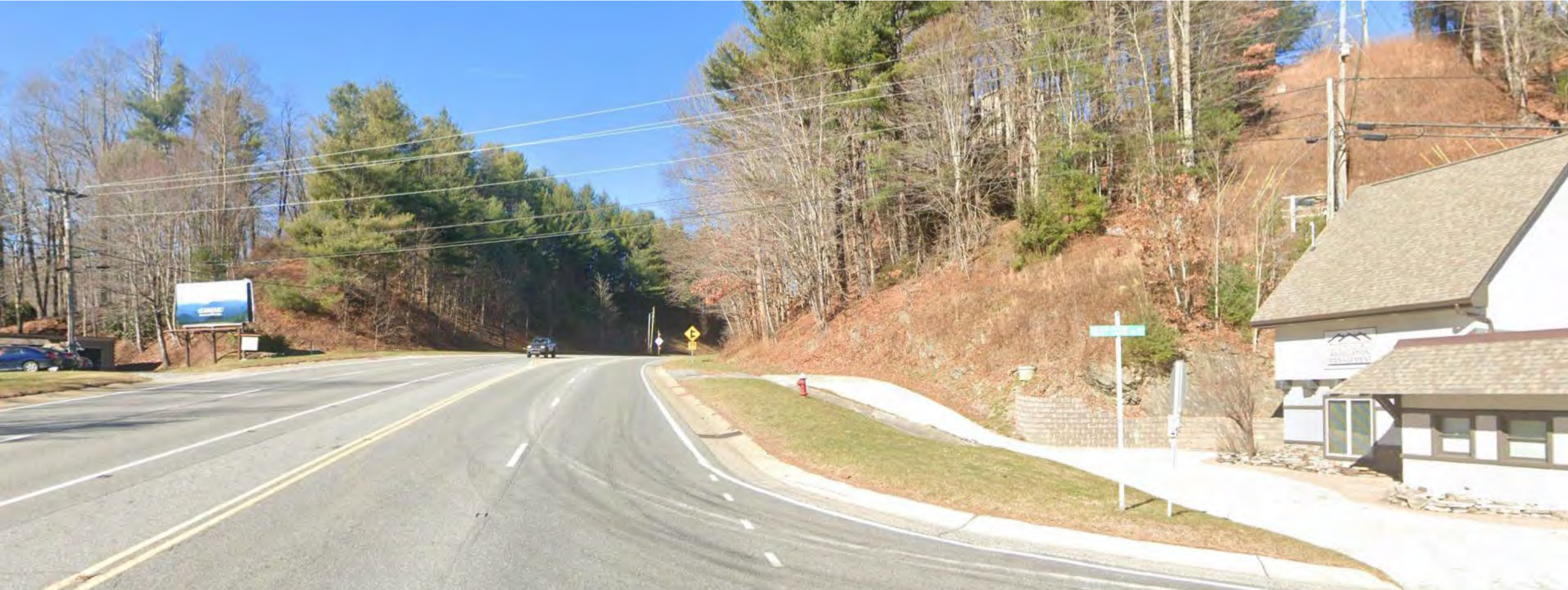
US 321 / Niley Cook Rd Intersection – Roadway Grade/Sight Distance/Traffic Speed, Utility Lines, Possible Pedestrian Bridge (Facing North)
