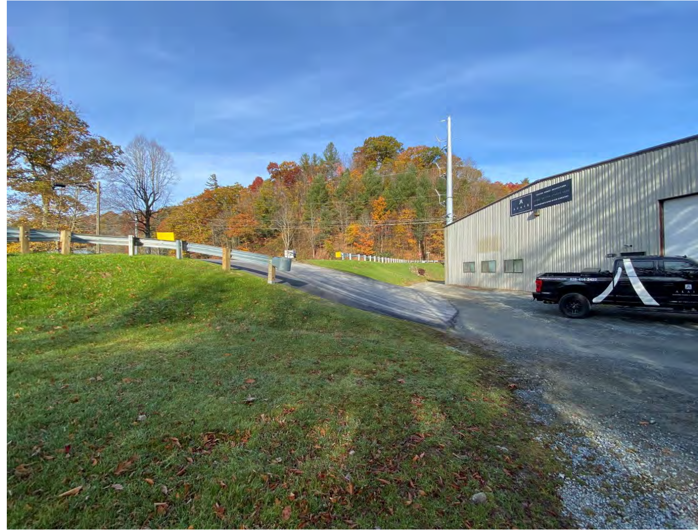
Steep Entrance Grade on North Side of Aho Rd Underpass
