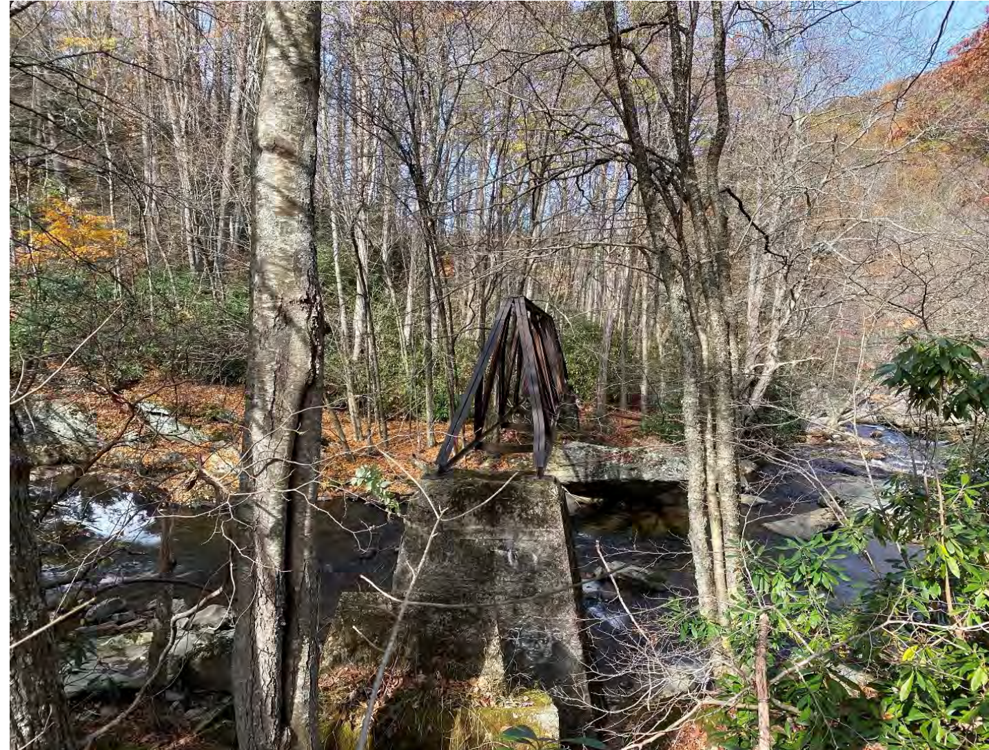
Abandoned Aerial Utility Crossing Over River – Possible Pedestrian Bridge Crossing Near this Location (Facing North Towards Future Boone Gorge Park)
