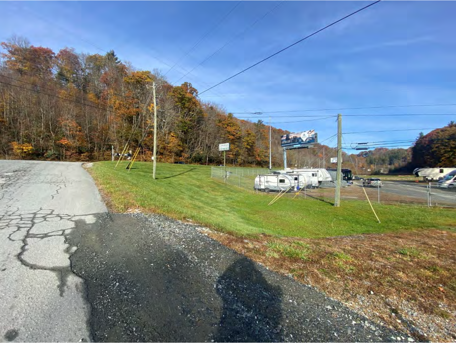
Roadway Embankment + Utility Lines + RV Storage Site (Facing West on Mack Hampton Rd)
