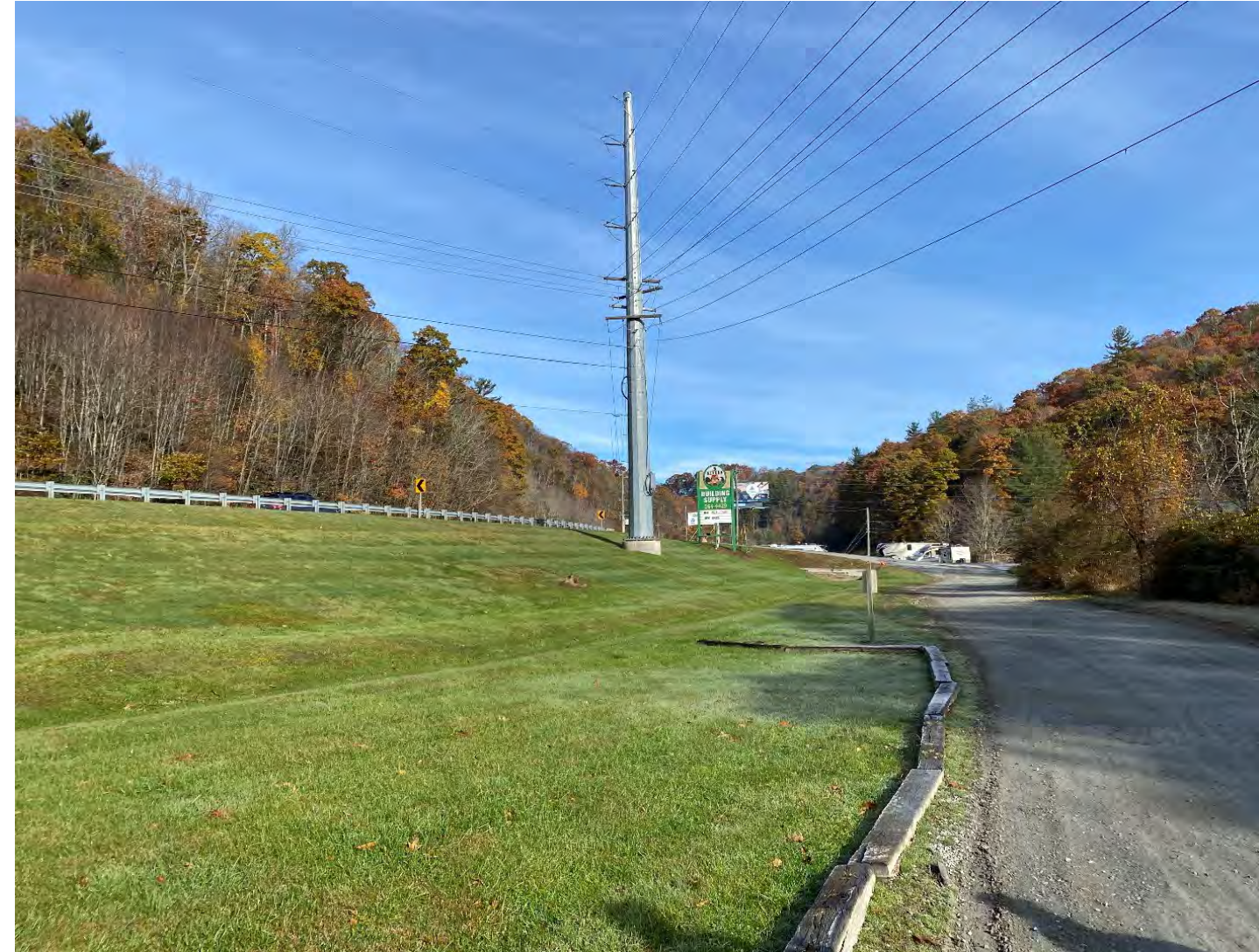
US 321 Roadway Embankment + Utility Lines (Facing North Toward Mack Hampton Rd)
