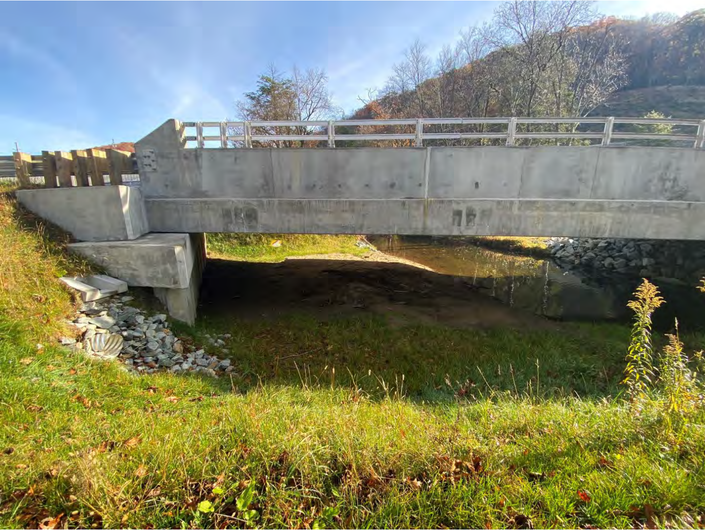
Aho Rd Underpass (Facing North)
